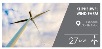
The 27 MW Klipheuwel Wind Farm is located in the Western Cape. The wind farm consists of 9 x 3 MW turbines which generates approximately 86 GWh per year, supplying enough electricity to meet the annual needs of more than 25,600 average South African homes. Globeleq is the majority shareholder and is responsible for asset management, operations and maintenance of the plant.
