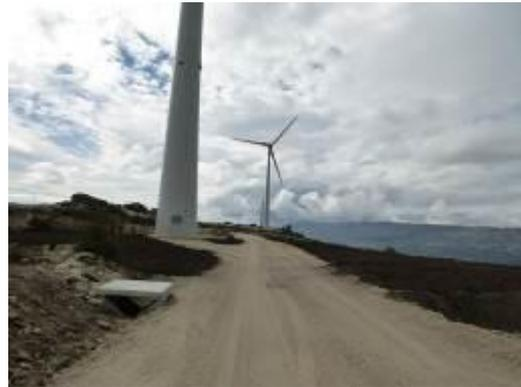
Photos 6.13 and 6.14 - Working platform adjacent to a wind turbine, on the left during the assembly phase and on the right after landscaping
