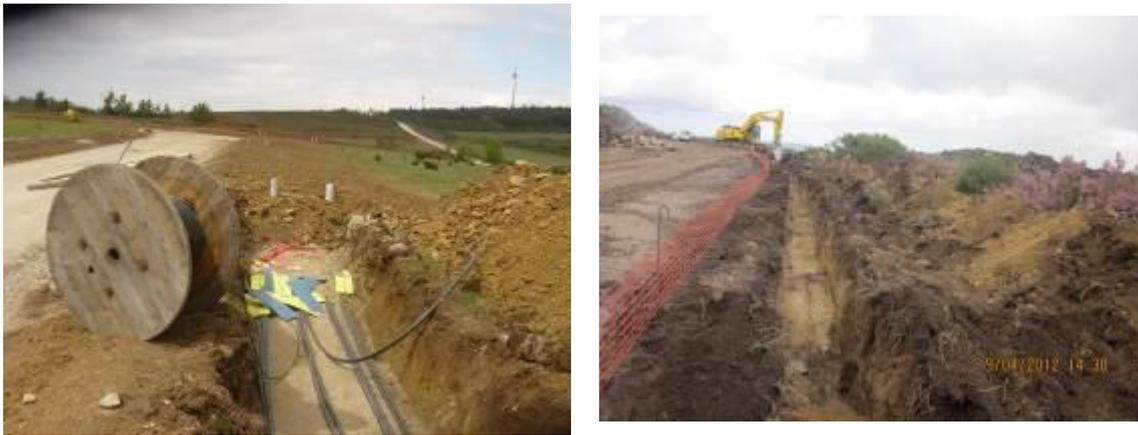
Photos 6.5 and 6.6 - Example of trench for electrical cable installation.
