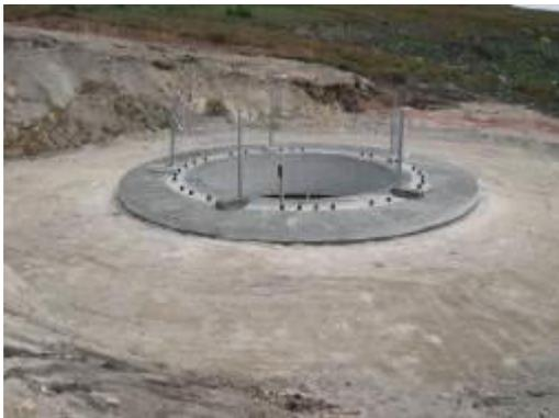
Photos 6.7 to 6.12 - Example of wind turbine tower foundation execution.
