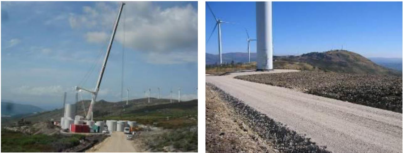
Photographs 4.5 and 4.6 - Example of working platform adjacent to a wind turbine, on the left during the assembly phase and on the right after landscaping
