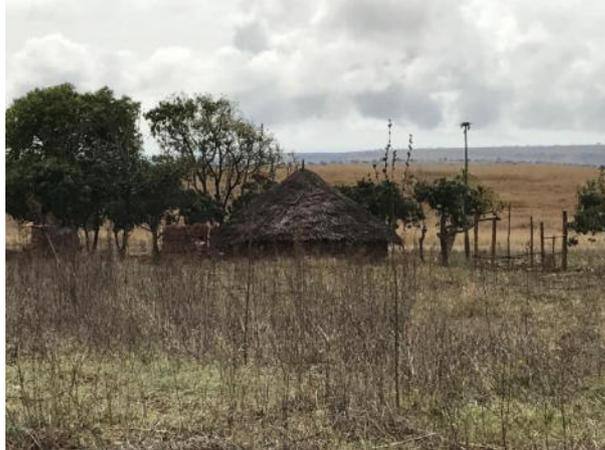
Photo 7.55 - Example of a house in Namaacha District with roof and walls made of reed/bamboo/palm trees
