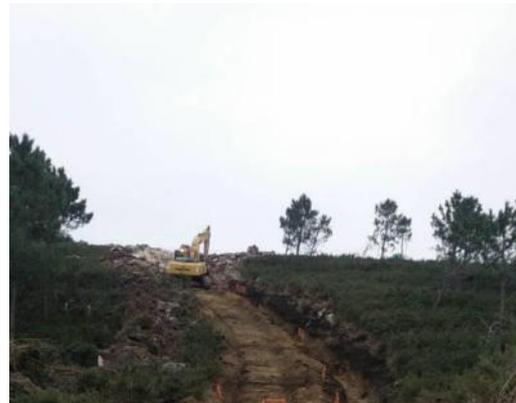
Photos 9.1 and 9.2 - Example of cable trenching along an existing access (left) and in natural ground (right)
