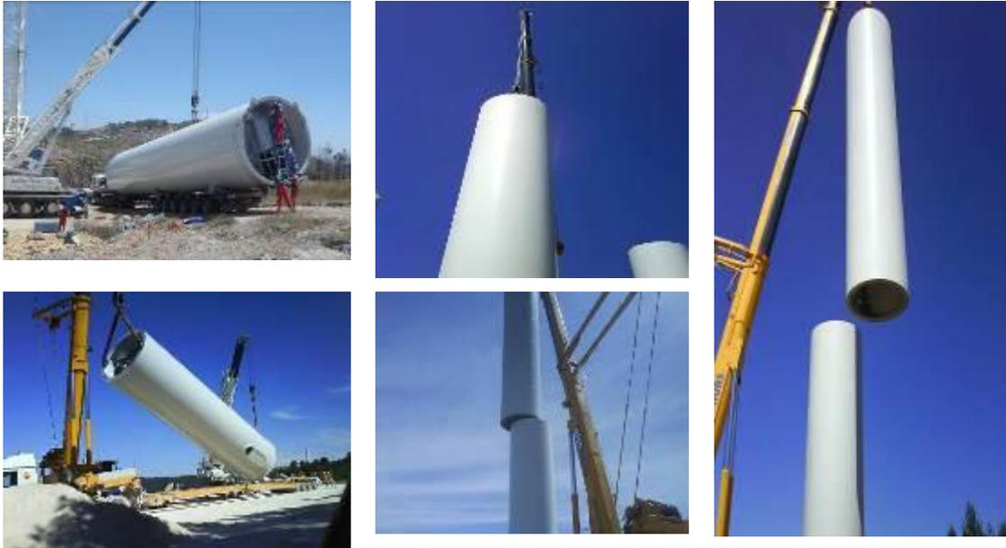
Photos 6.17 to 6.21 - Example of wind turbine tower assembly
