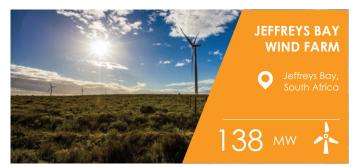
Jeffreys Bay Wind Farm in the Eastern Cape has an installed capacity of 138 MW, with 60 x 2.3 MW turbines generating approximately 448 GWh annually. The electricity is exported into the national grid, and Globeleq is the majority shareholder responsible for asset management, the balance of plant operations, and maintenance. The plant generates enough electricity to meet the needs of 114,100 average South African homes.
